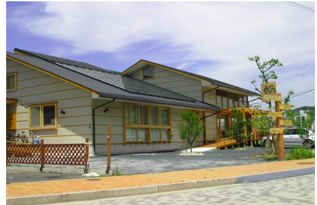
Recently constructed ecological office building Kitikyushu with simplified “OM Solar” roof mounted active air collector supplying thermal mass storage for heating and cooling.
